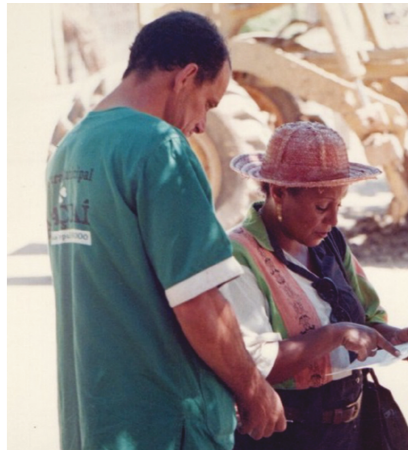
Maria evaluating and discussing with a municipal worker at a construction site. Araçuaí, 1998.
